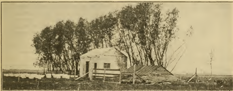
FIG. 7.—E. G. Brown's upground cellar constructed by setting four fence posts about four feet into ground at the four corners of the proposed cellar. The portion of the posts above ground are boarded up on the outside. The dirt on the inside is shoveled out, forming an embankment around the board fence. The whole is covered with a roof as shown.
